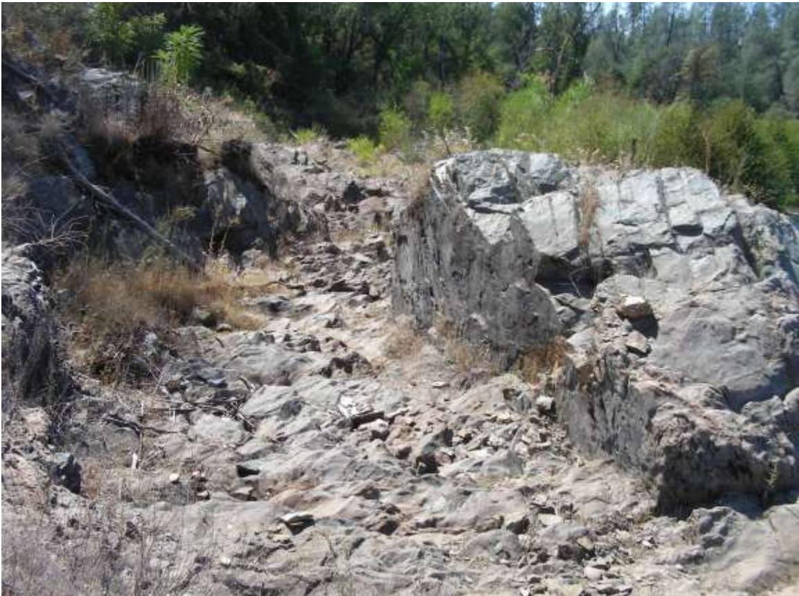
Site of the old fish ladder at Saeltzer Dam along Clear Creek Road. The ladder was needed when the older Taylor Dam was raised about ten feet.
