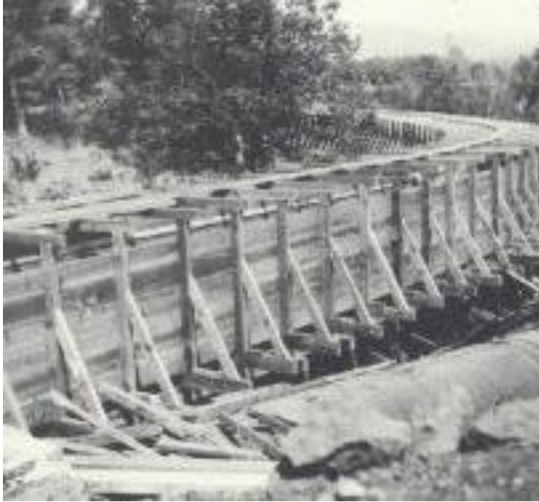
Northern California Power Company flume being built as part of the Battle Creek Project. Courtesy of Shasta Historical Society.
