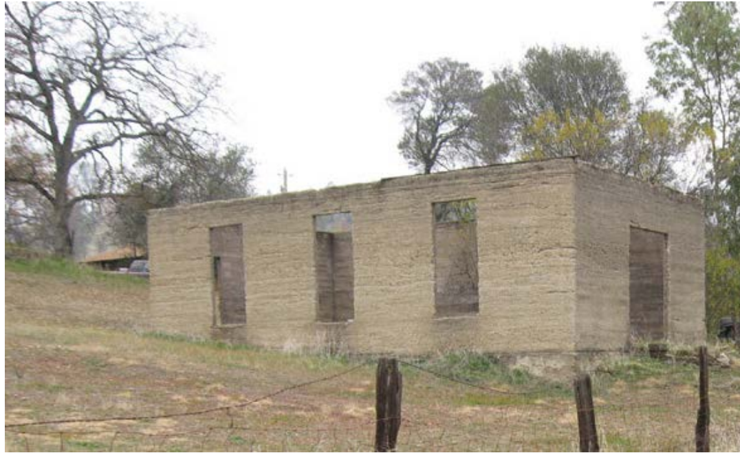
Richland Baptist Church on Church Street in Ono.
